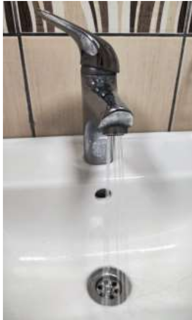
The use of perlator in water taps
